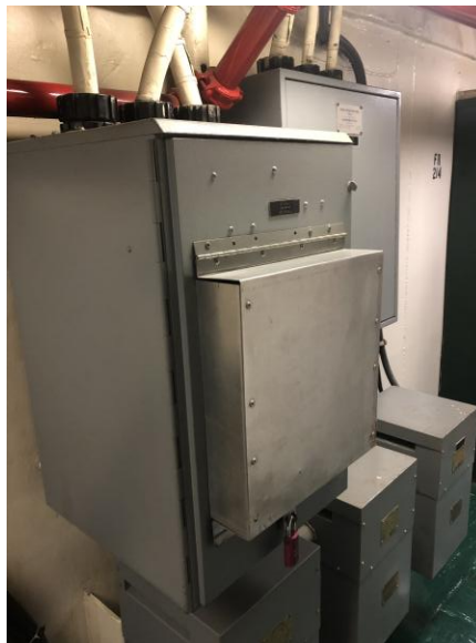
Figure 3: Automatic Bus Transfer (© 2022 by Norbert Doerry)
